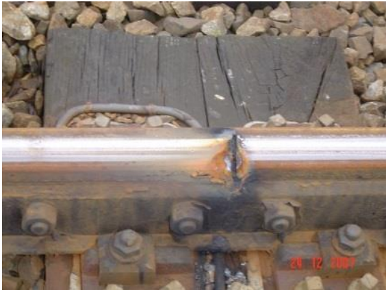
Burned insulated joint
